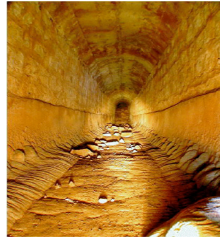
Carbonate deposits in the aqueduct channel of the Fréjus Roman aqueduct, France
